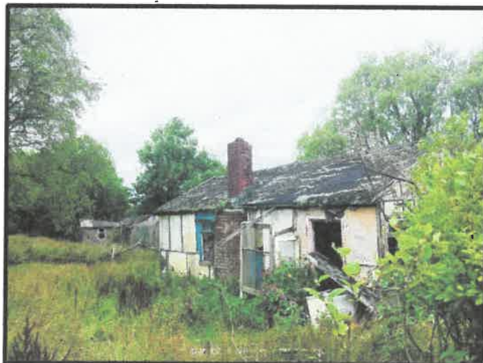
Derelict Bungalow - Chinatown
