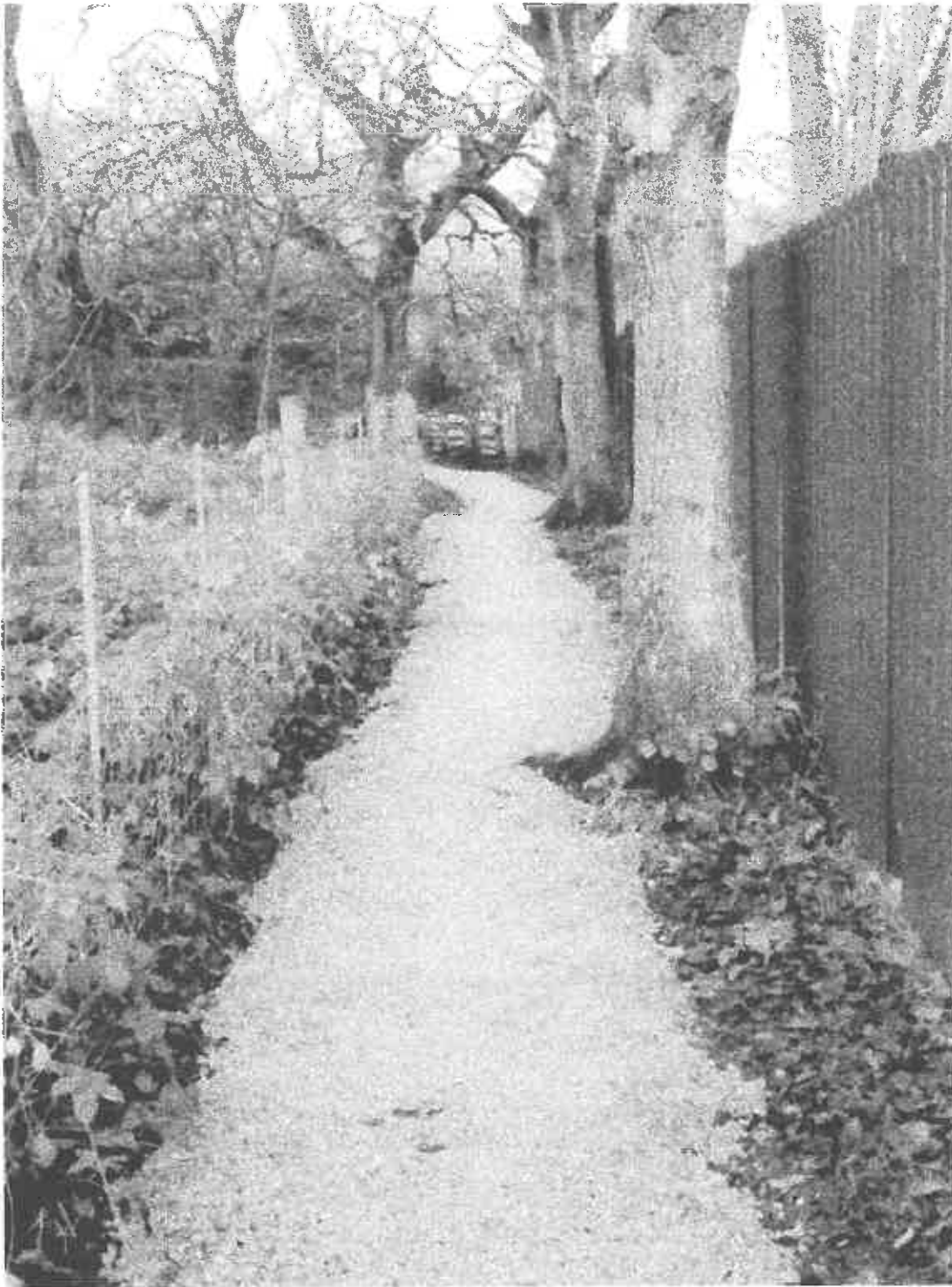
Footpath 16-after improvement
