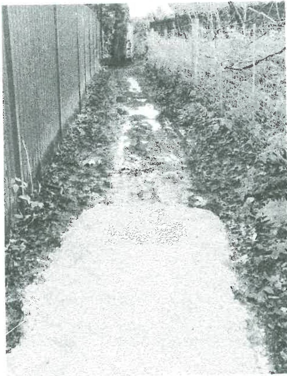
Footpath 16-the work in progress
